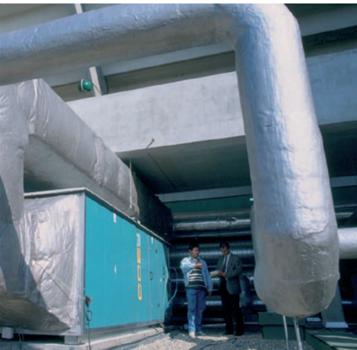
Circulating pumps for building management
